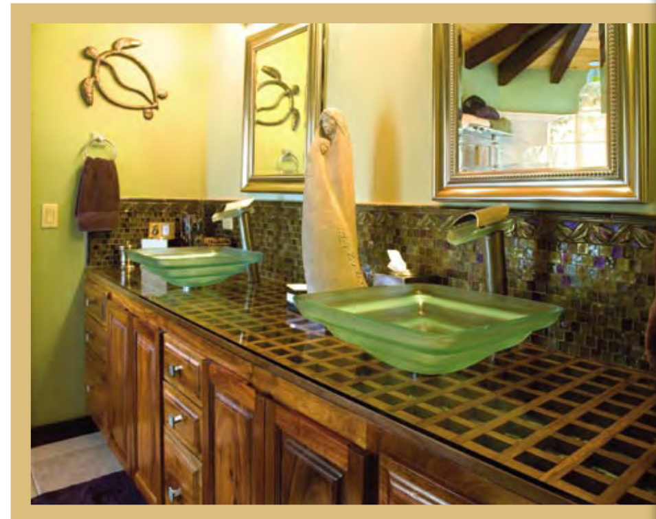
John topped his handcrafted koa cabinets with an ohia lattice counter and a glass top. Beneath the ohia is copper sheeting distressed for a patina effect. Sparkling backsplash tile and trim are from Bella Pietra.
